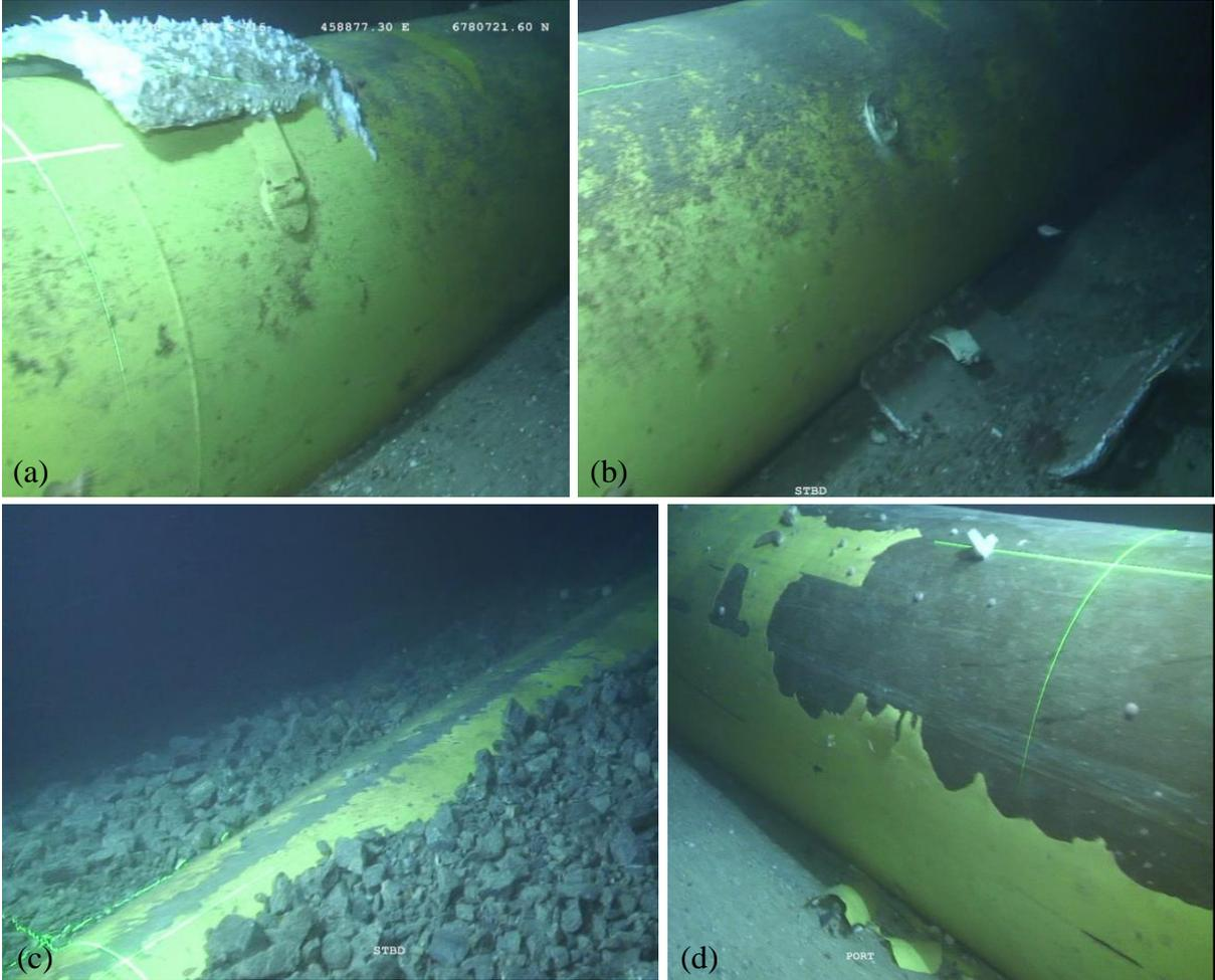
*Figure 1. Trawl damage to bundles: (a) slightly deformed anode, otherwise intact, (b) anode ripped off and located next to bundle, (c) coating scraped off on top of bundle and (d) extensive coating removal around bundle circumference*
